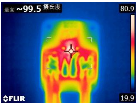
Package Thermography (Input Current 40A)
