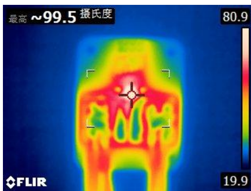
Package Thermography (Input Current 40A)
