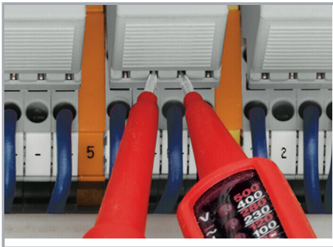
Function testing via touch-proof test slots
