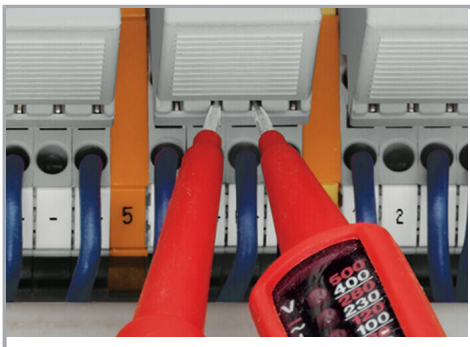
Function testing via touch-proof test slots
