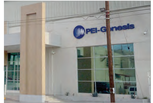
Production Facility, Nogales, MX
