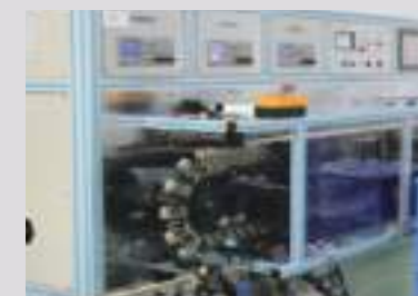
Automatic electrical test workshop
